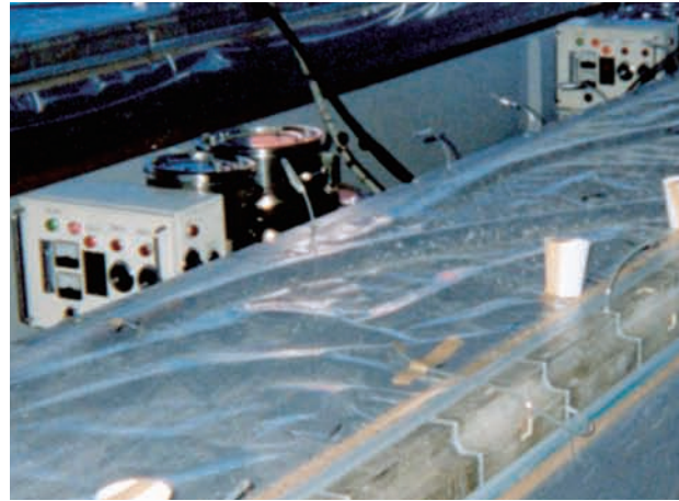
(10) 裏込注入材(U-グラウト)注入
