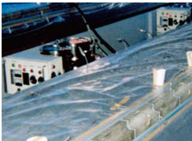
(10) 裏込注入材(U-グラウト)注入
