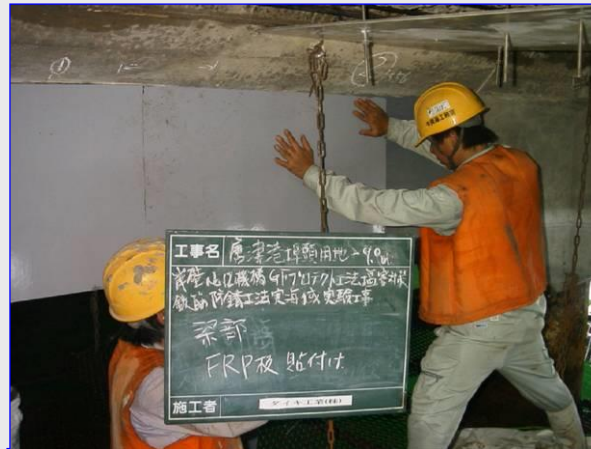
FRP Sticking repair
