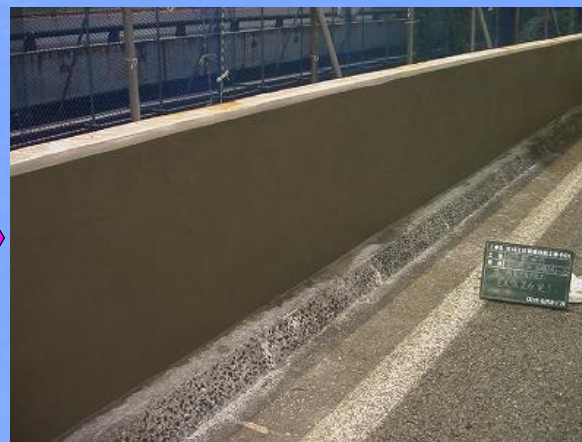
SLUG LEAD # 100 # 450 Salinity countermeasure mortar is done
