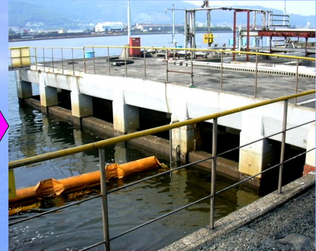
Seven years after completion
