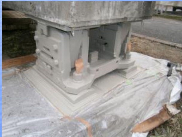
After undercoat application
