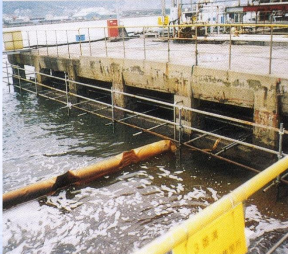
Before construction (Overall picture)
