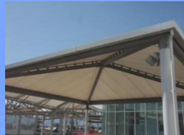
Two years after construction
