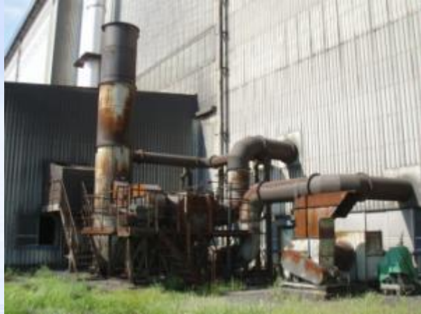
NYB Outdoor Exhaust Facility Before construction
