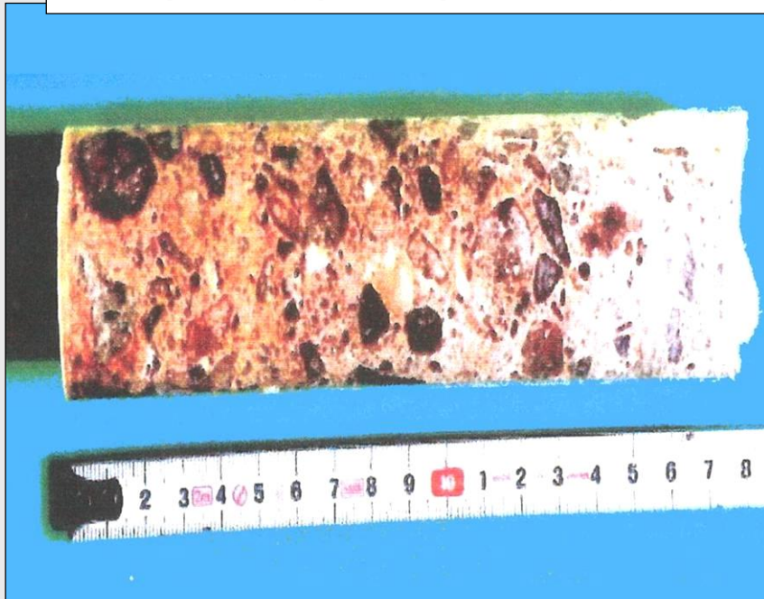
Expressway pier Expiration 10 years
