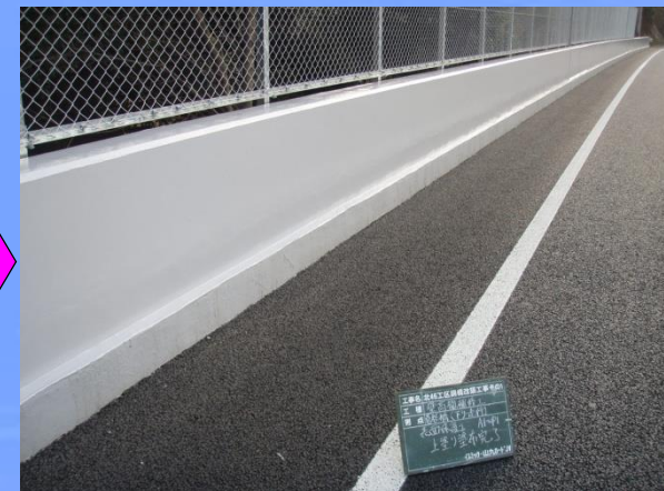
Surface protective coating B specification complete
