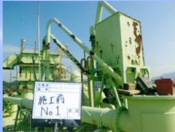
Cement silos Before construction
