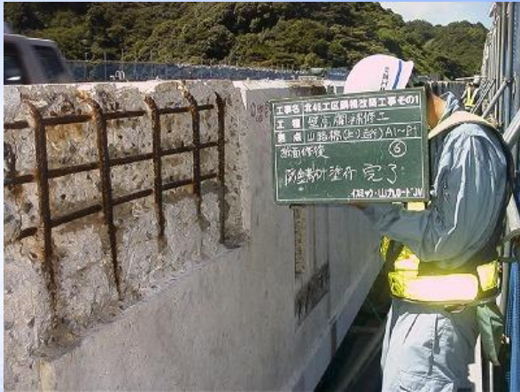
Rebar rust preventive agent SLUG LEAD # 100 Application
