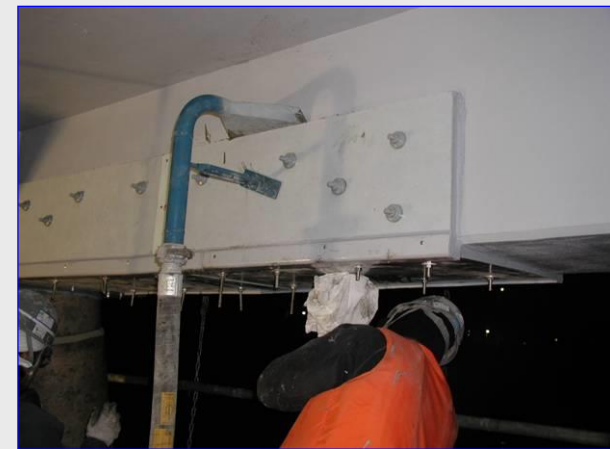
Grout injection by injector
