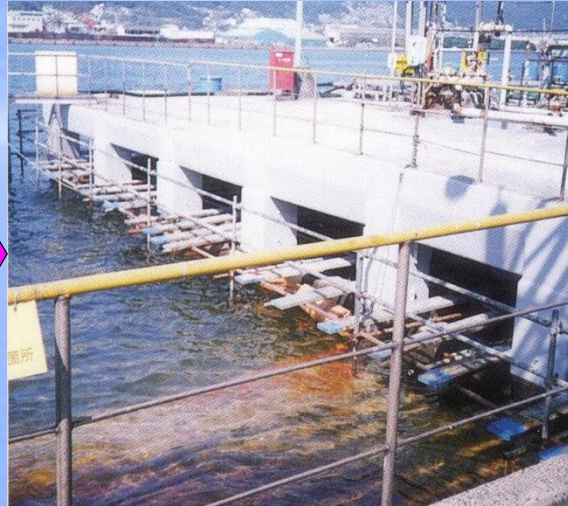
Immediately after completion
