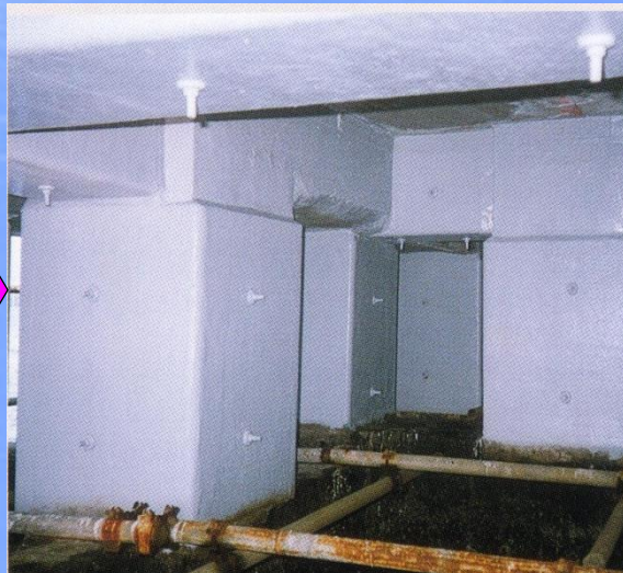
Immediately after completion
