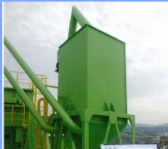
Cement silos After construction
