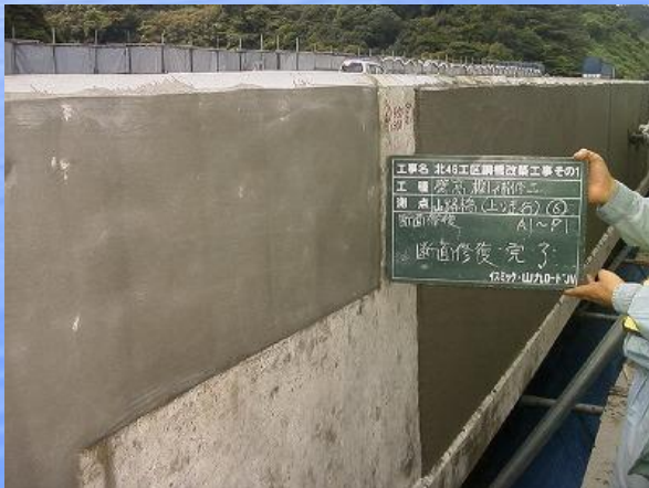
cross section Repair completed
