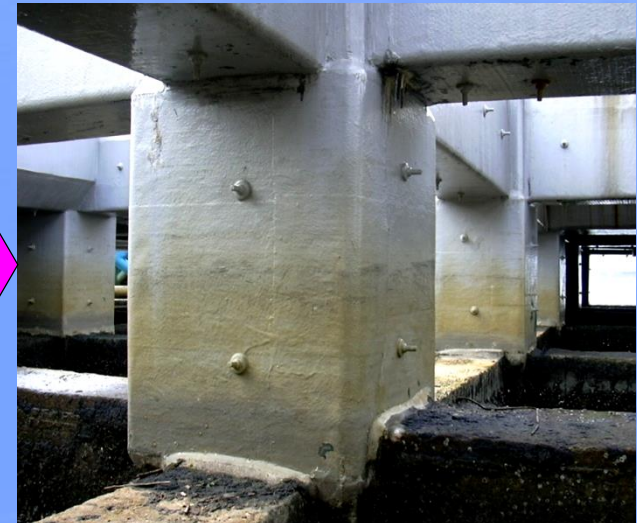
Seven years after completion
