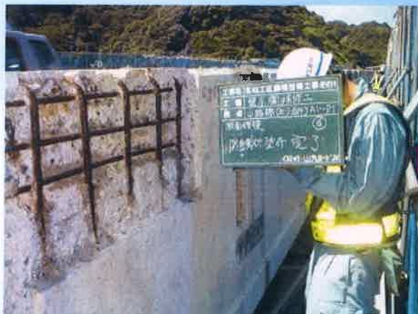
塗佈鋼筋防鏽劑Slag Lead #100
