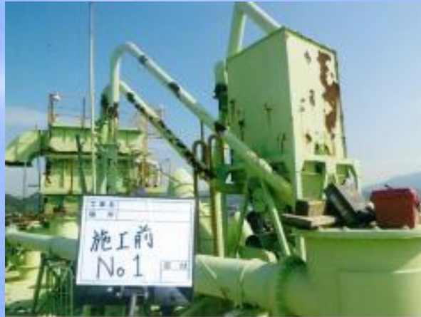
Cement silos Before construction
