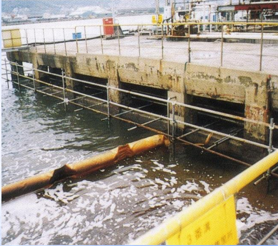
Before construction (Overall picture)
