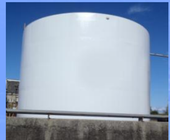
Chemical factory After construction
