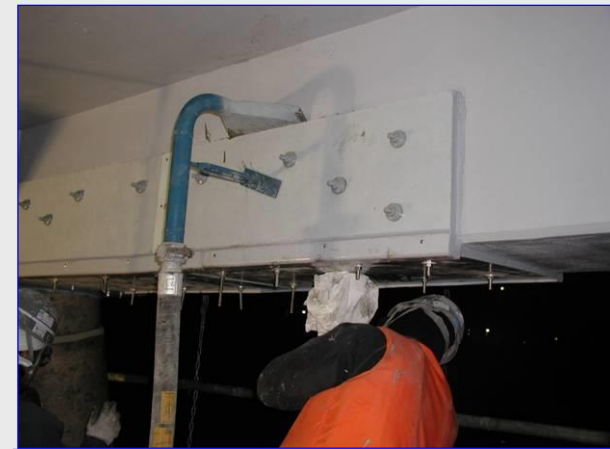
Grout injection by injector
