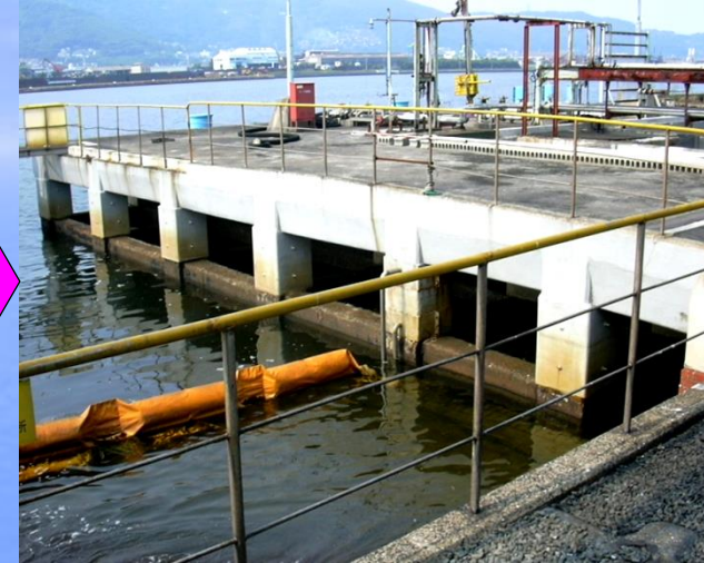
Seven years after completion
