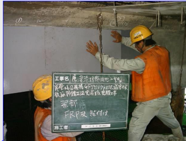
FRP Sticking repair
