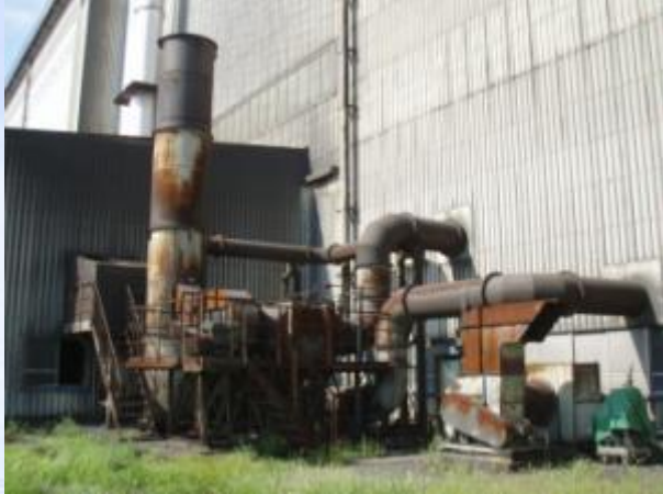
NYB Outdoor Exhaust Facility Before construction
