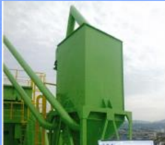
Cement silos After construction
