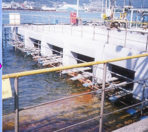
Immediately after completion
