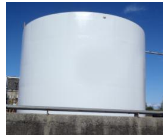
Chemical factory after construction
