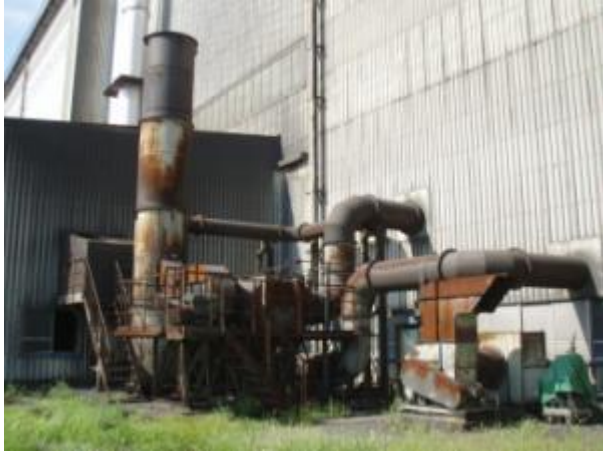
NYB outdoor exhaust equipment before construction
