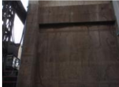
Concrete wall surface
