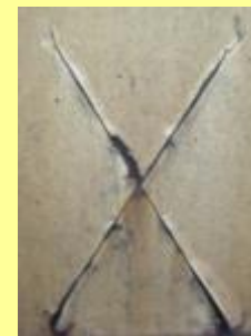
SlagLead SR 2 deterioration
