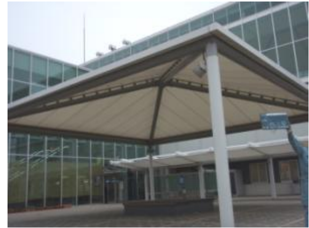
Right after construction
