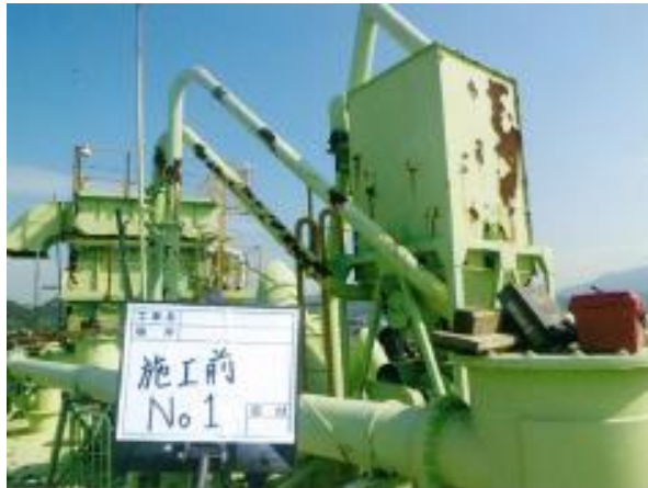
Cement silo before construction
