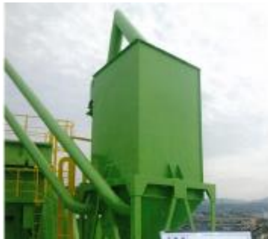
Cement silo after construction
